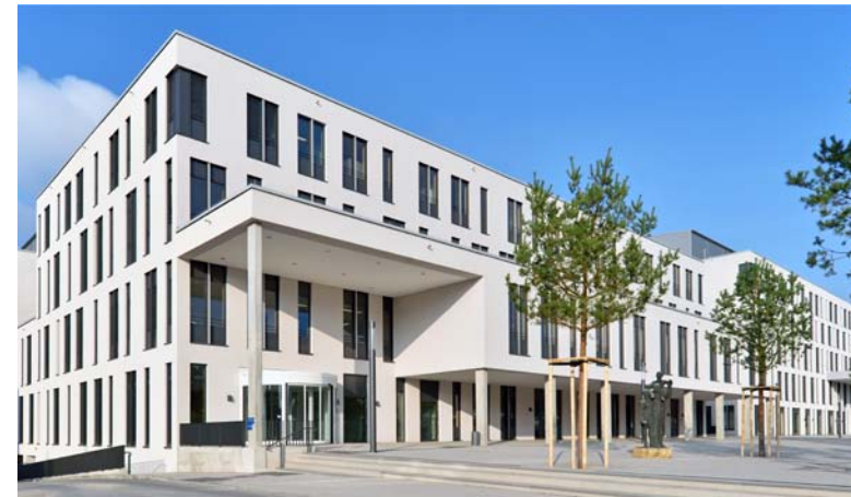
Fig.: Houses E and A (right) of the new clinical complex.
